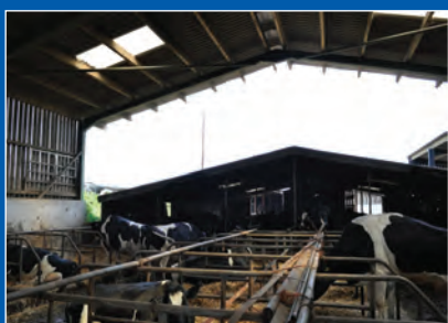
The cattle shed has been extended, with an increased roof height for better ventilation
