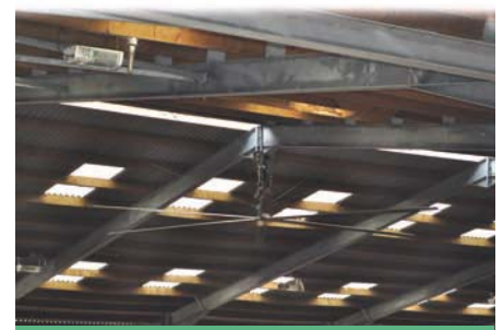
Ventilation from overhead fans allows cattle of all ages to be housed under the one roof
